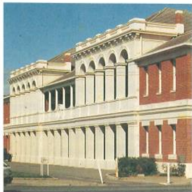
Courthouse Buildings, Marine Terrace (Built 1897)
