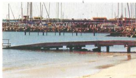
One of three small boat launching ramps - Town beach
