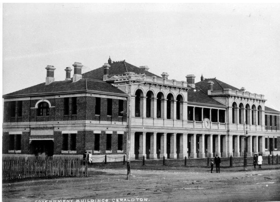
Government Buildings (Geraldton Courthouse), Marine Terrace, Geraldton, c1900. Image donated by A.C. Burns, P 1571
