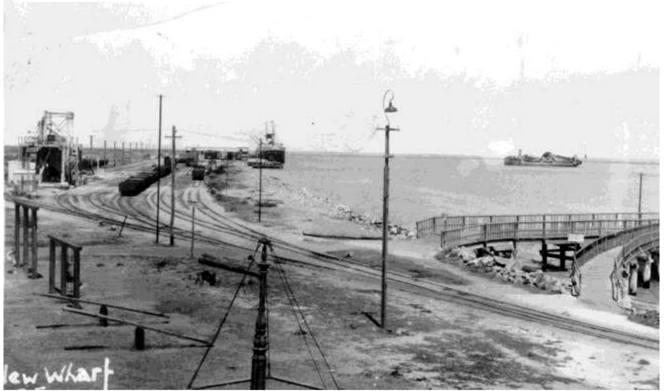
P 924 CONCRETE WHARF. DREDGE SIR WILLIAM MATTHEWS AND ESPLANADE JETTY 1931
