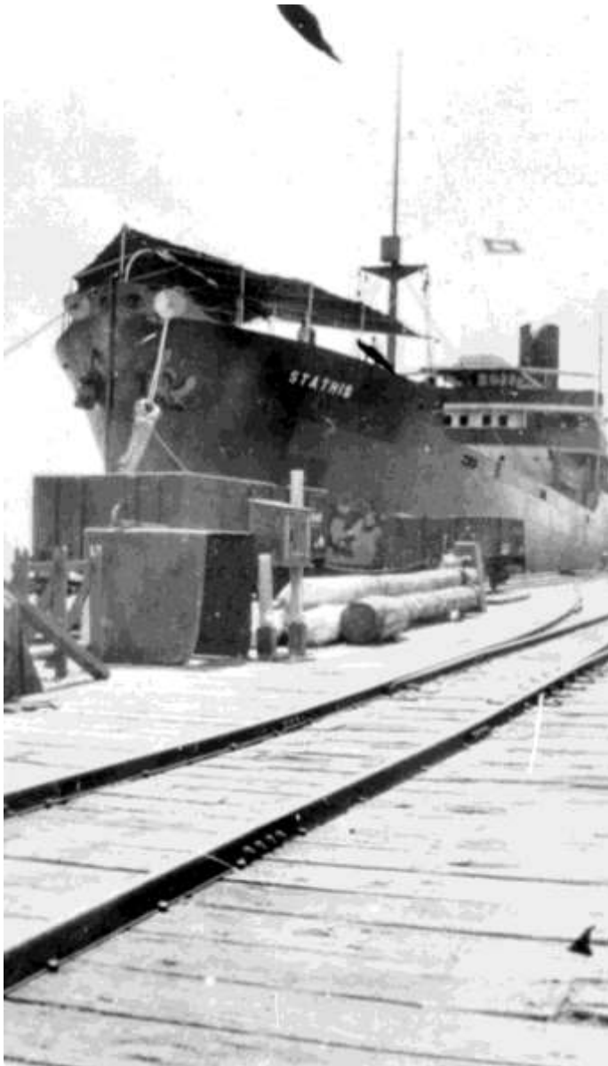
P 765 SHIPS ALONGSIDE RAILWAY JETTY
