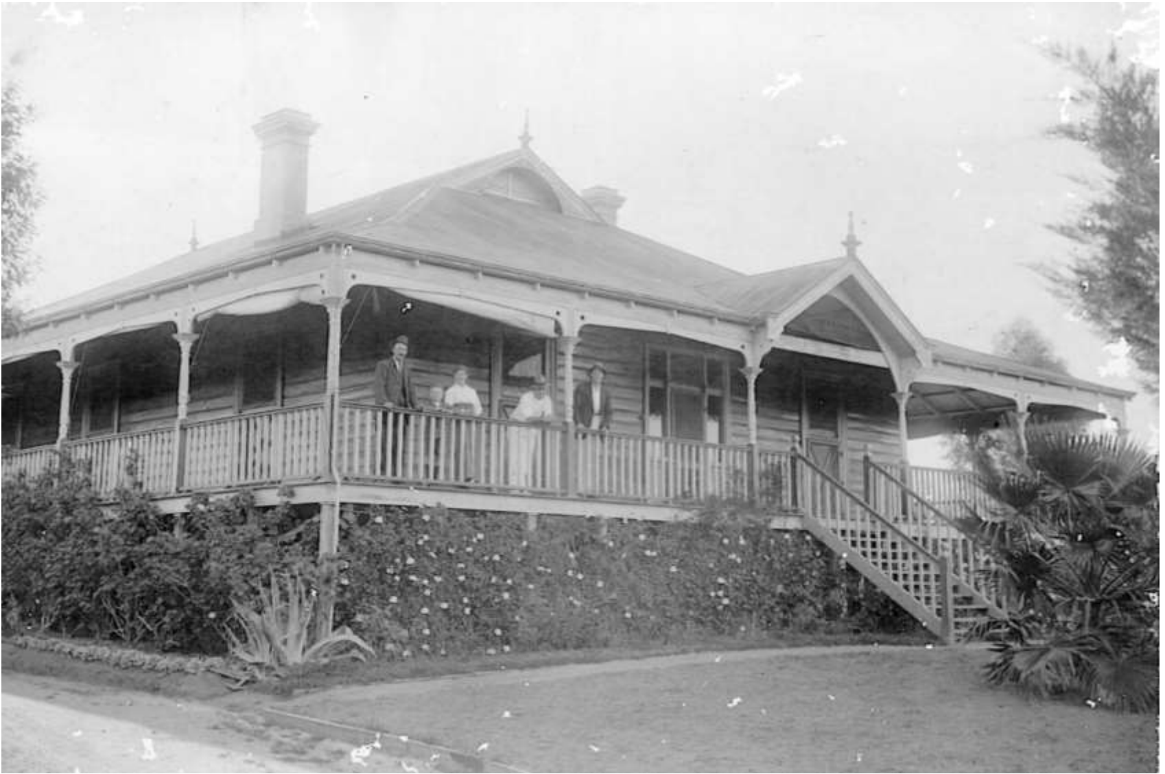
820: MINE MANAGERS HOUSE PROTHEROE LEAD MINE c1922/23
