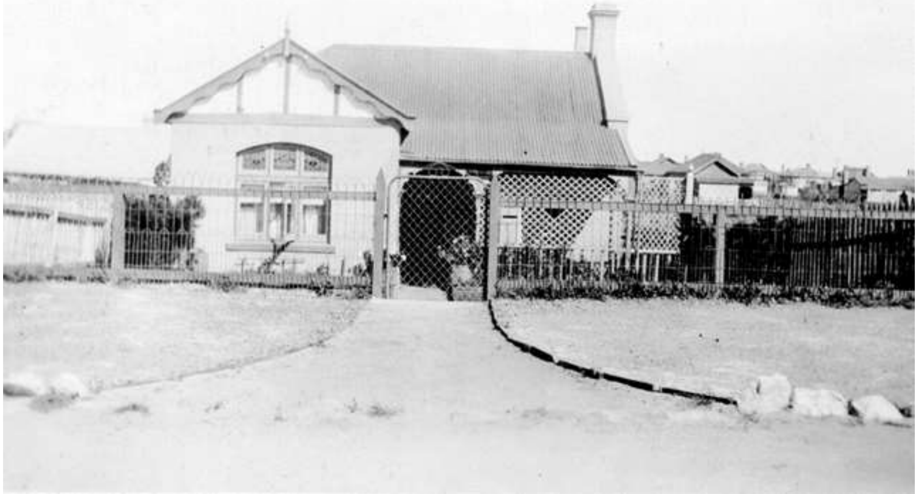
142: BELIEVED TO BE 9 CONWAY STREET GERALDTON HOME OF BOB AND EILEEN SCAMP. WAS BUILT BY EILEEN'S FATHER HENRY JOSEPH WATSON
