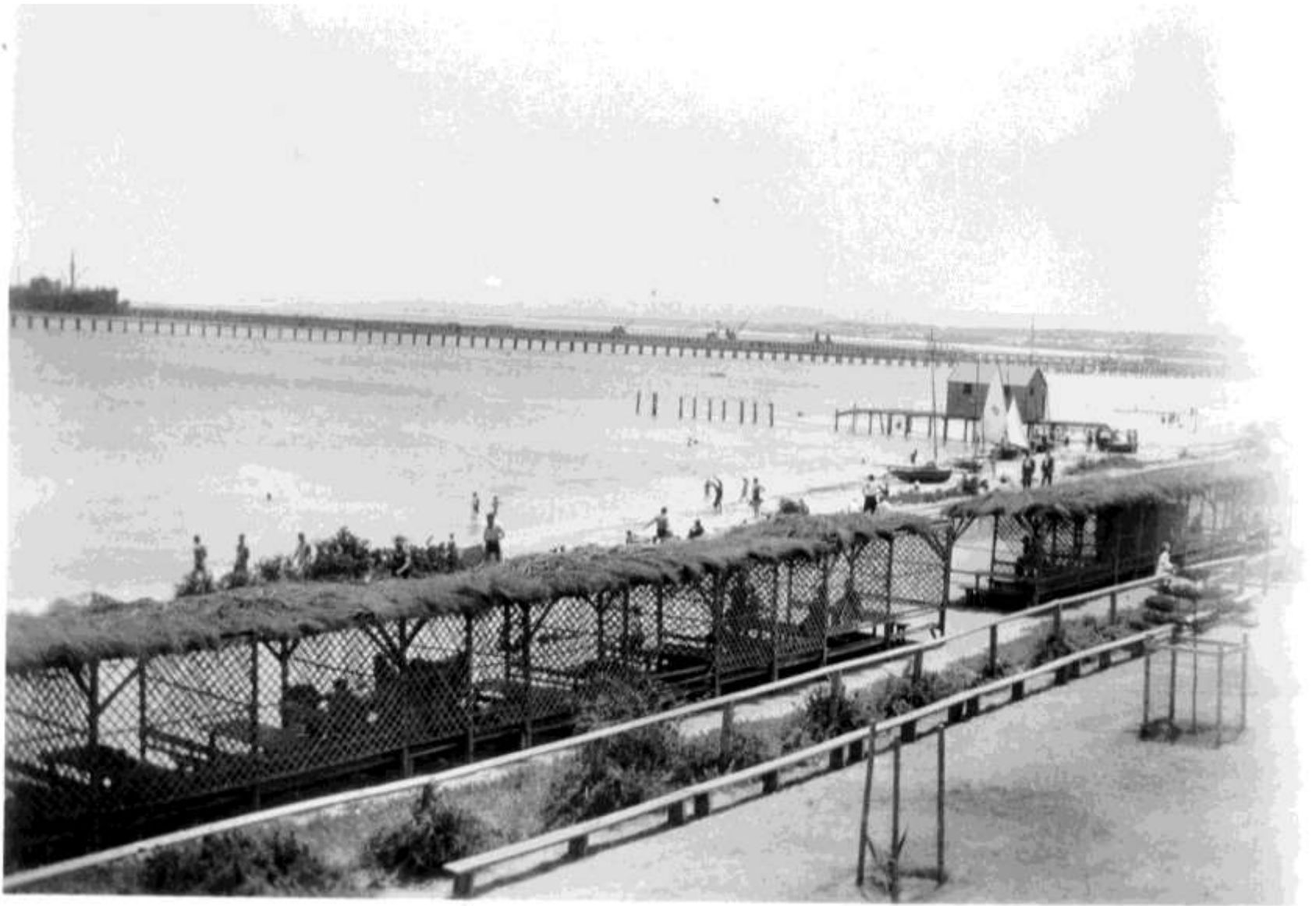
797: SHELTER SHEDS COVERED IN TEA-TREE BRUSHING WITH LATTICE ON GERALDTON'S ESPLANADE BEACH c1920s
